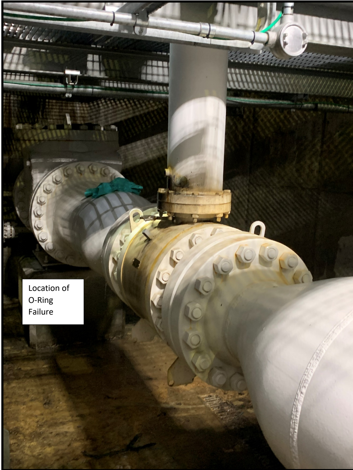
Photo 6 —looking west at 20-inch valve from within the containment area after clean-out.
