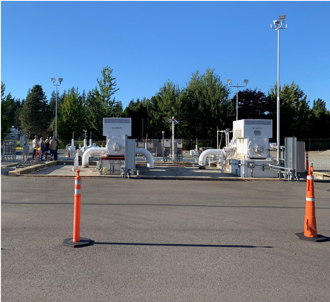
Photo 2 —looking north across 20-inch valve location and containment area.
