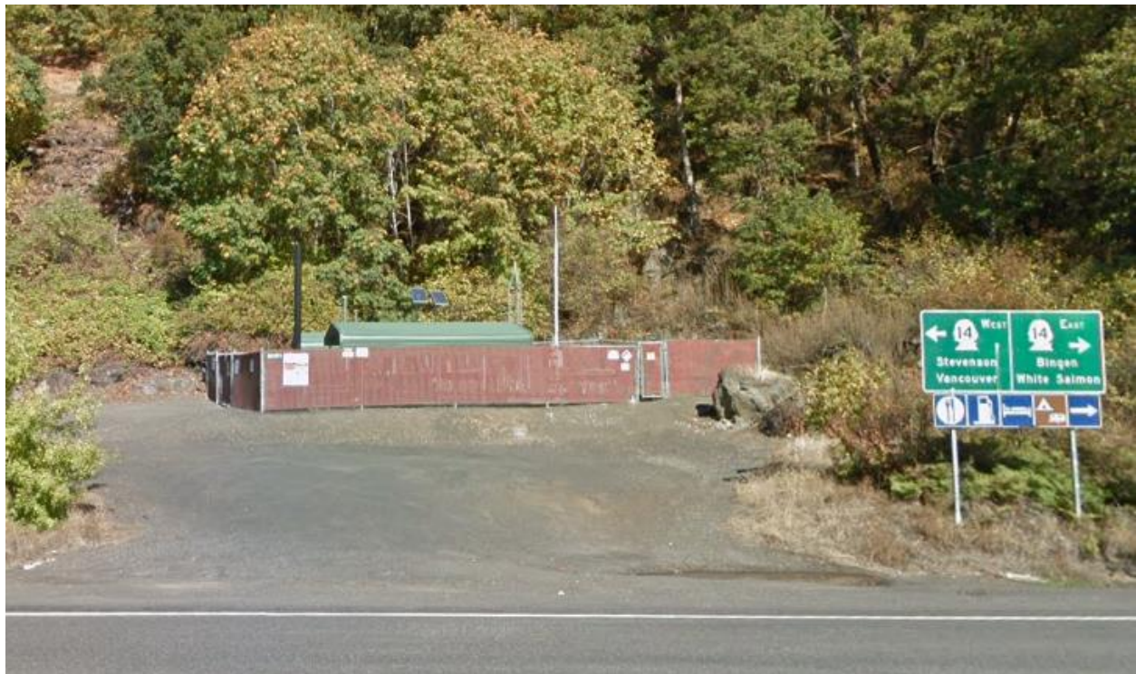
Figure 2: Street View of Hood River Meter Station Before Damage
