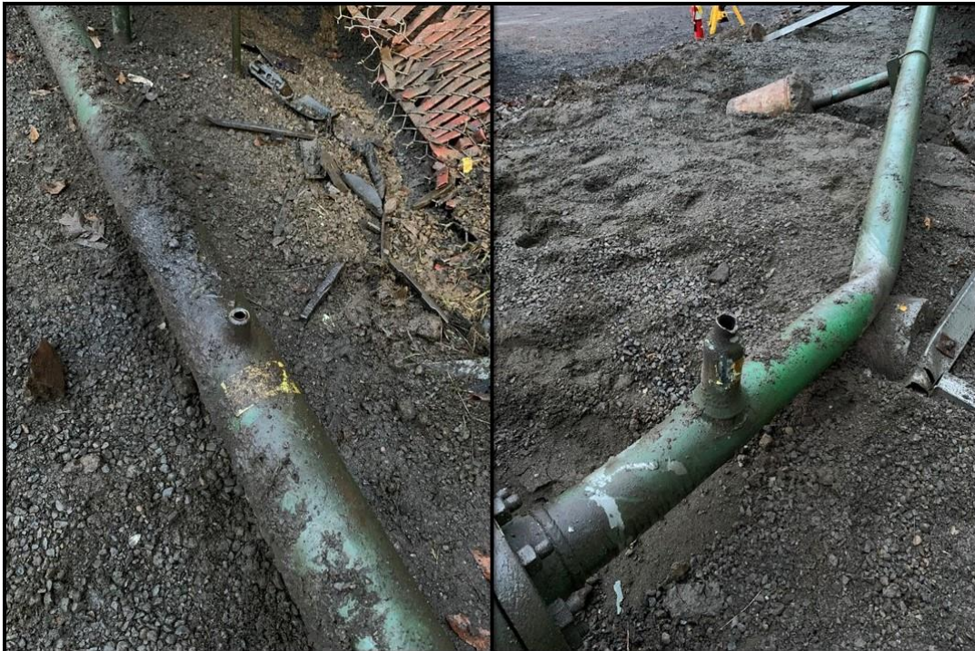
Figure 6: Close up photo of leak locations.
