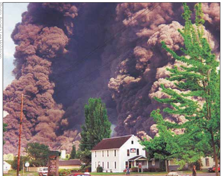
1999 failure of a hazardous liquid pipeline in Bellingham, WA
