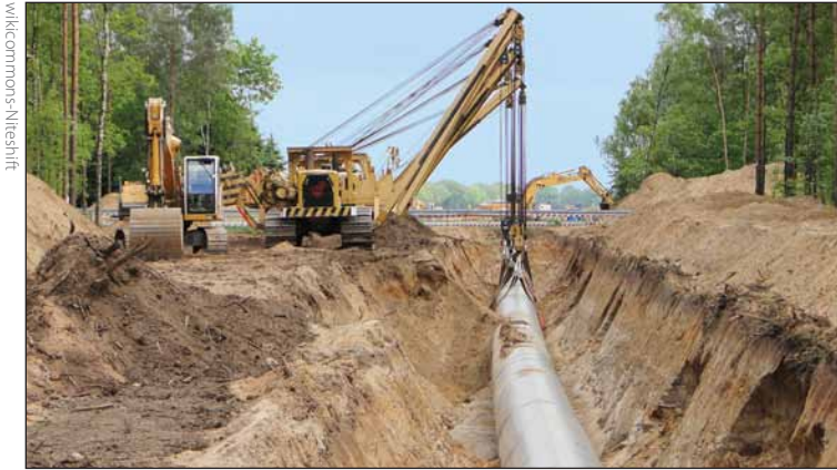
Construction of Gas Transmission Pipeline
