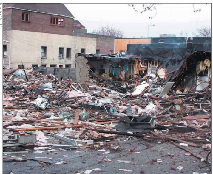
2016 explosion from a gas distribution pipeline in Seattle, WA
