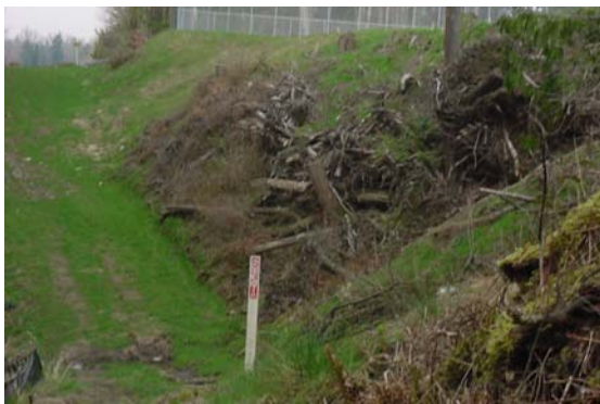
Figure 5 – Retention pond near easement
