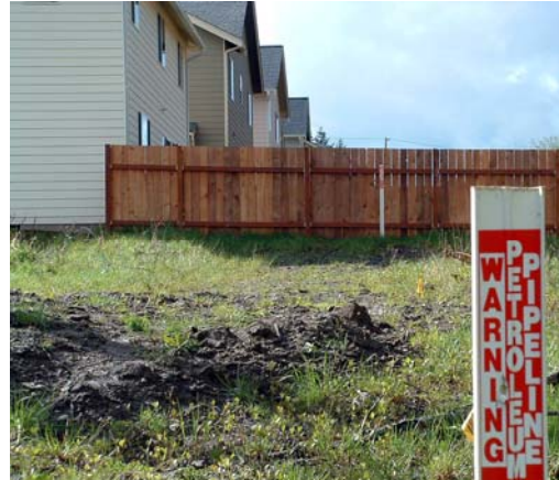
Figure 4 – Fence on pipeline easement
