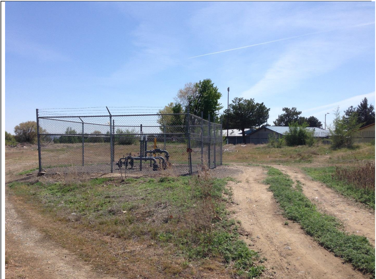
Looking East-note closest structures are approximately 100 ft south.
