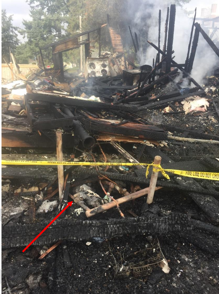
Figure 2 – View of the damaged two-meter manifold covered in debris
