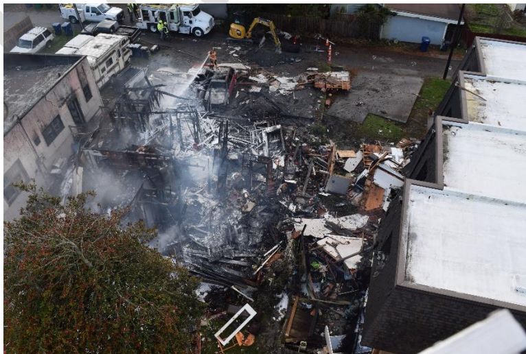
Figure 1 – Aerial view of the duplex following the explosion. Image provided by MVFD
