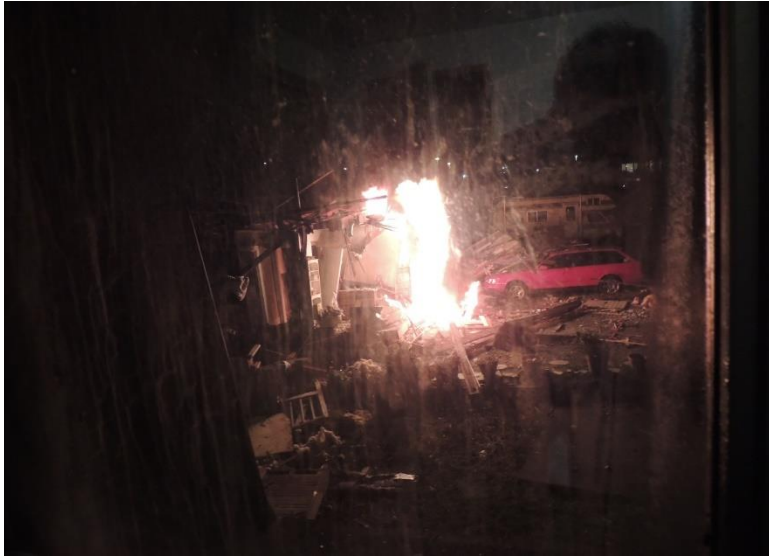
Figure 3 – Fire being fed by the gas meter shortly after the explosion. Picture taken by neighbor, Corban Gassaway
