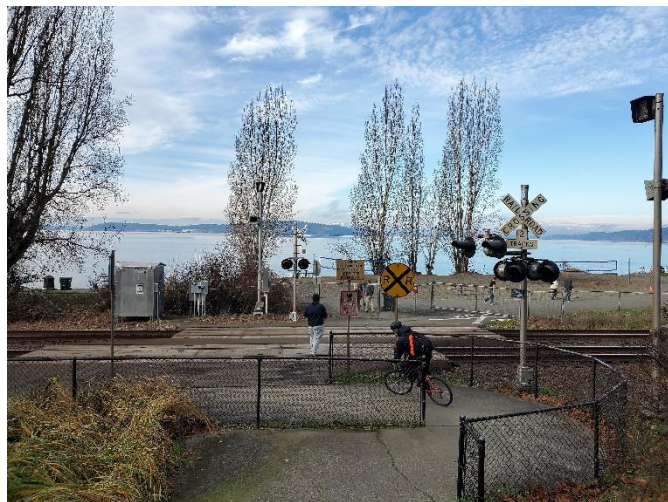
Figure A-3: Z Channelization at Sunnyside Beach (USDOT 085754X) Steilacoom, WA
