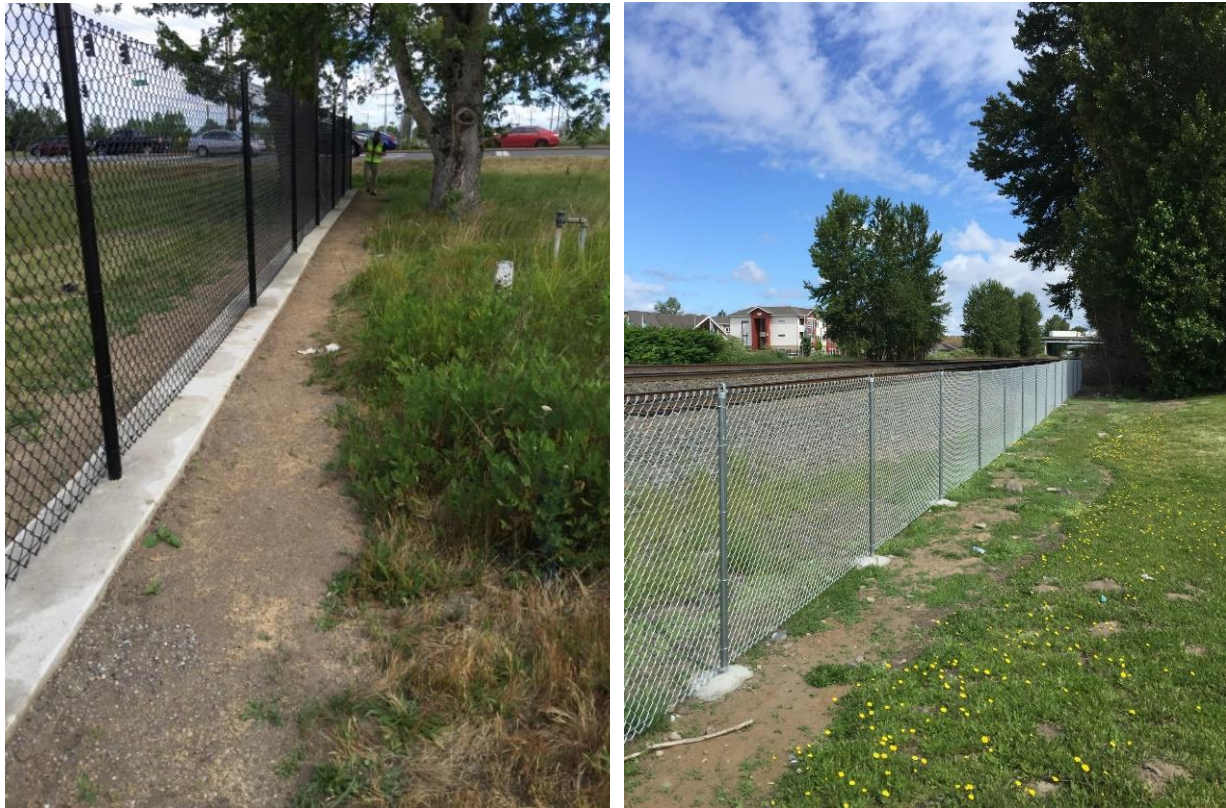
Figure 25: Fencing Project in Kent, WA, to Deter Trespassing
