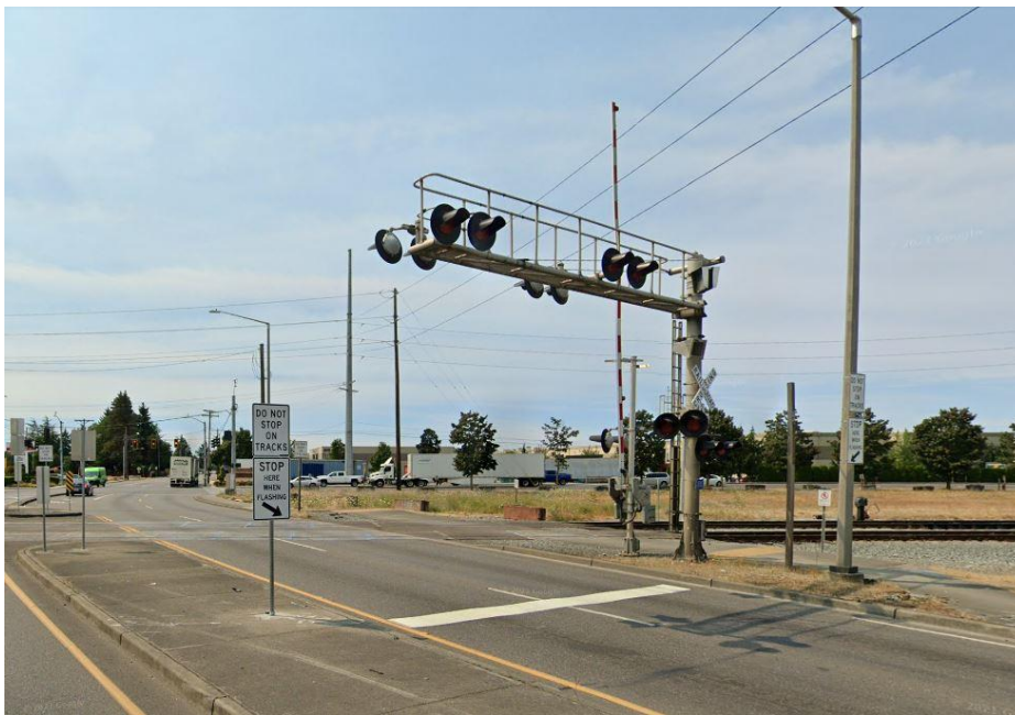
Figure A-11: Example of Wide Raised Median 100th Street SW (USDOT 085402S) in Lakewood, WA
