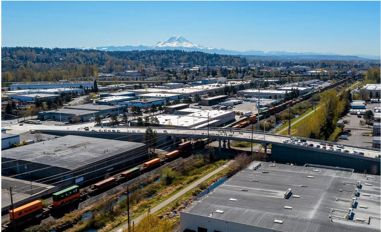
Figure 22: FMSIB Project #35 Kent, Washington – S. 228th Grade Separation (USDOT 085627W)
