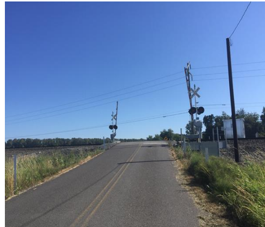
48th Avenue NW – After installation of active warning devices. (Source: UTC.)
