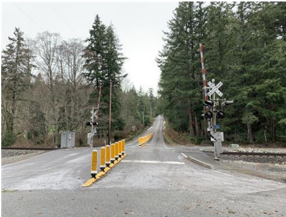
Figure A-12: Delineators at Cove Road (USDOT 084795Y) in Whatcom County, WA
