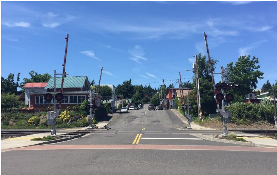
Figure A-9: Example of Right-angle Four-quadrant Gate System at Russell Avenue (USDOT 090148C) in Stevenson, WA
