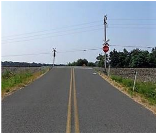
48th Avenue NW – Before installation of active warning devices. (Source: UTC.)
