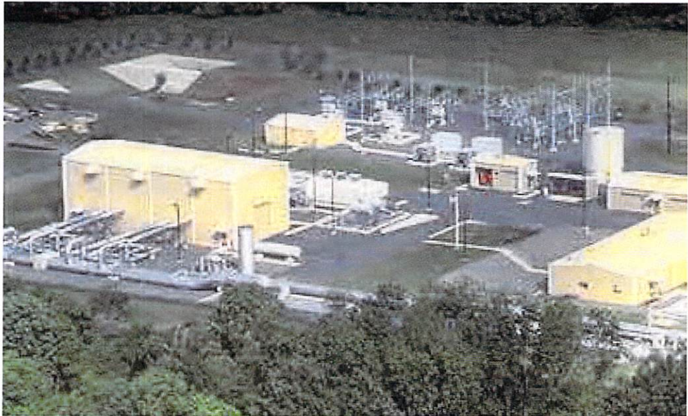
Gas transmission compressor station.
