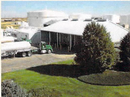
Truck loading facility.
